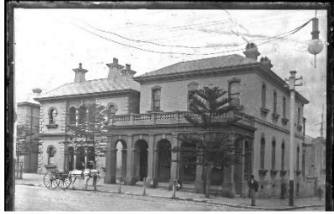
Newcastle Post and Telegraph Office, Hunter and Watt Street
